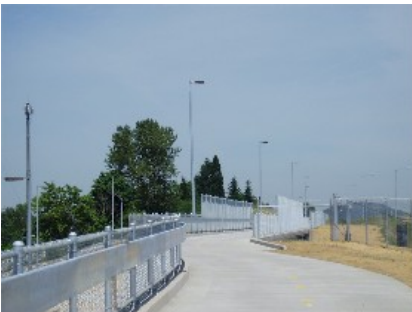
The completed overpass over Powell Boulevard
