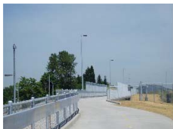
The completed overpass over Powell Boulevard
