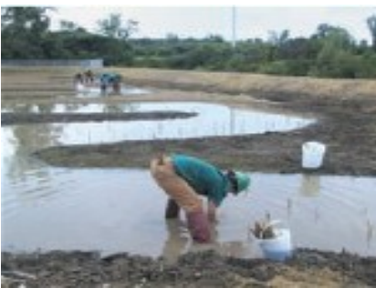
Restoration of Bartlett Brook
