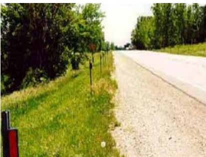
Strieter-Lite reflectors line local road
