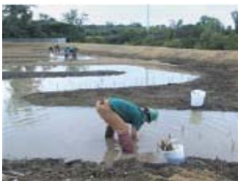
Restoration of Bartlett Brook
