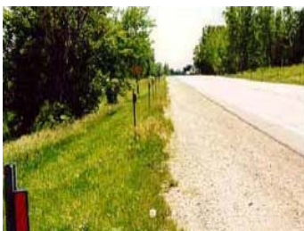
Strieter-Lite reflectors line local road
