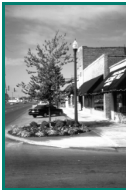
Figure 3: Broadway at 8th after TE improvements, (looking west).
