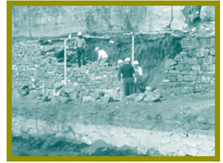
Workers rebuild Georgetown wall using dry-stone masonry technique. (Photo: D.C. DPW)
