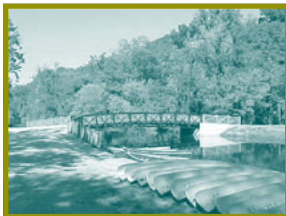
The new Fletcher's Boathouse bridge links people and vehicles with the popular canal towpath, a rail-trail, and the Potomac River. (Photo: D.C. DPW)
