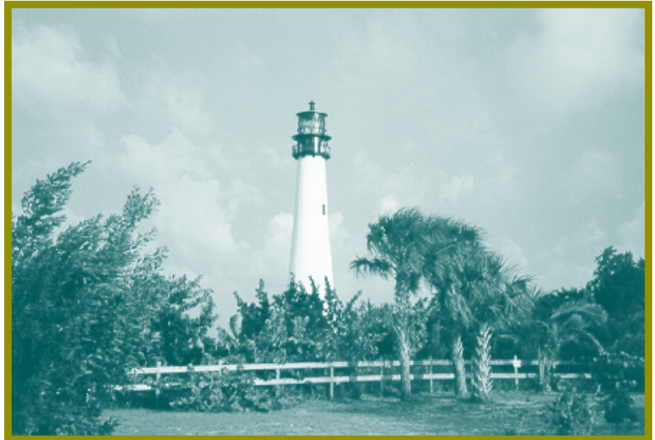
The restoration of Cape Florida Lighthouse in the Bill Baggs State Recreation Area was one of the first TE projects in Florida. (Photo: FDOT)
